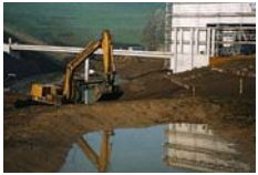
Infiltration swale under construction. Water started to accumulate here even in the building phase.
